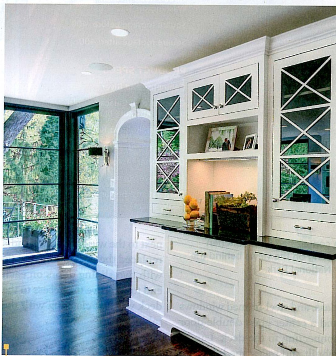
The team designed and fabricated custom cabinets with inset doors. White oak strip flooring is stained to match all of the flooring in the first level of the house.
